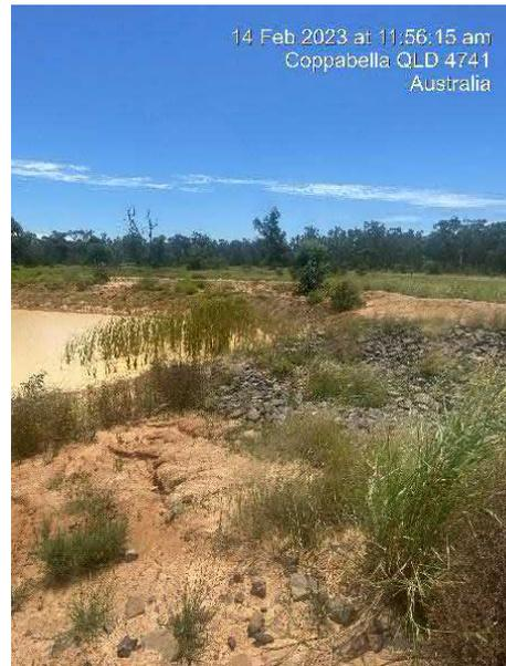
Drain condition and rock armouring IPEE southern sediment pond outlet – 1
